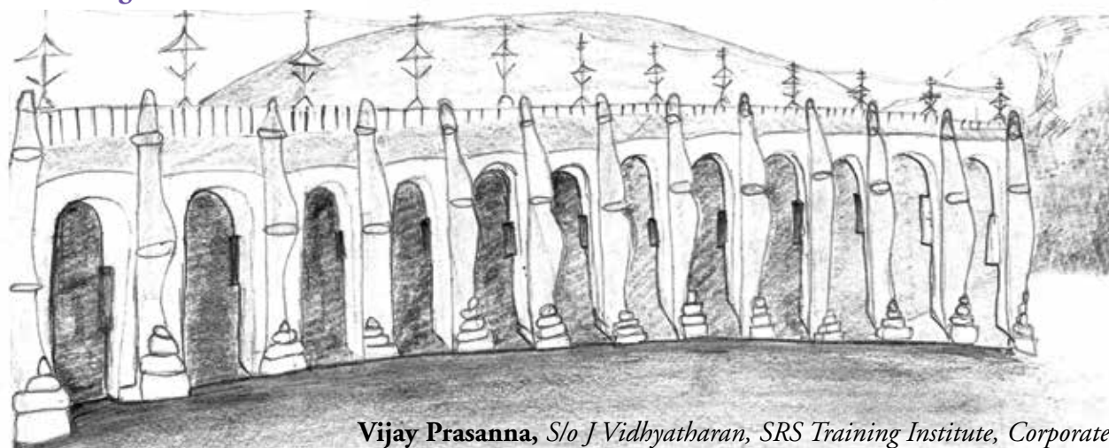
A view of 16 sluice gates of Mettur Dam
