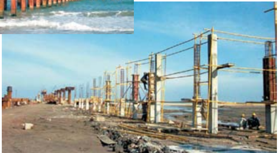
A view of the pipeline support structures.
